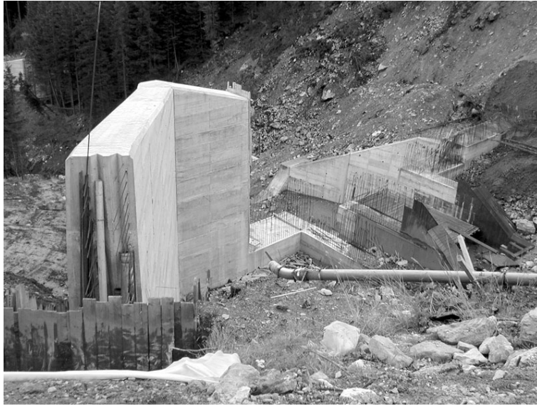
Figure 4. Retaining walls and debris-sorting dams are built along Blaubach torrent as a protective measure. Photograph taken October 23, 2000.
